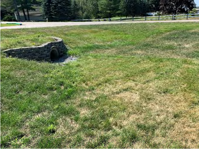
29 Gundalow -1 (Drainage Area)
