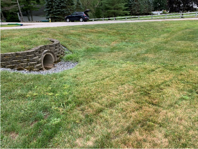
29 Gundalow -1 (Drainage Area)
