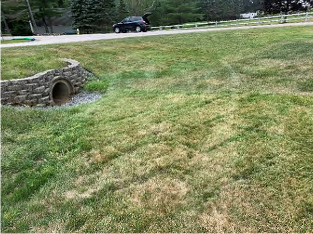
29 Gundalow - 1 (Drainage Area)
